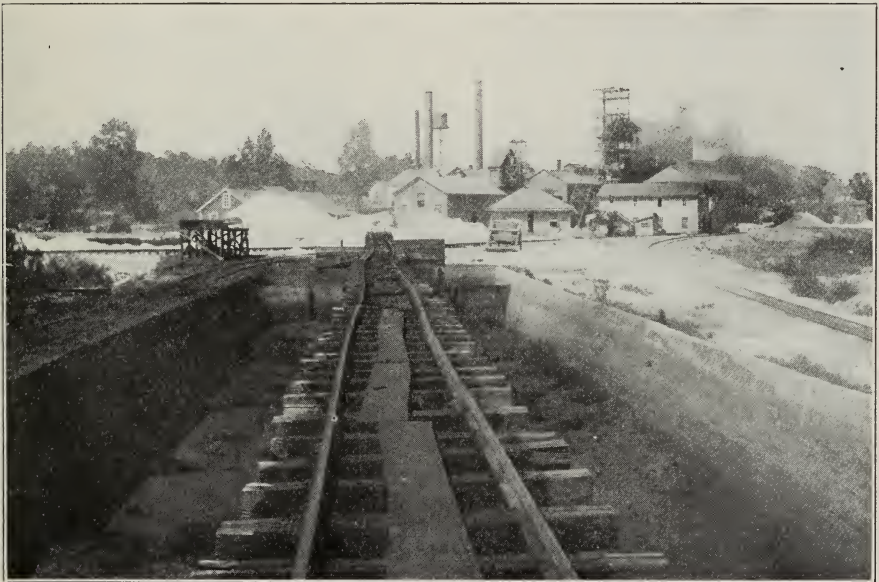
FIG. 41. Main shaft and mill of Rosiclare Lead and Fluorspar Mining Company.
